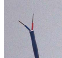
Stripped shielded wire with ground wire trimmed
